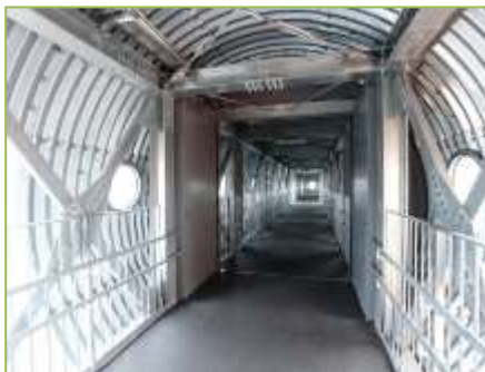
Boarding Bridge for passenger on foot at 2 nd floor
